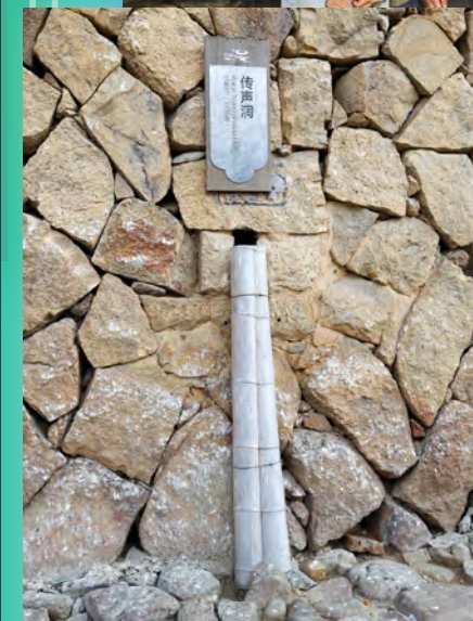
The ancient 'voice transmission hole', strategically, is used to amplify and transmit sounds, allowing inhabitants to communicate across large spaces without raising their voices.
